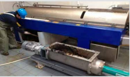
In the seaweed extract application, the NETZSCH pump was installed with a custom flanged hopper to connect to the centrifuge discharge, which conveys the end product into totes.
