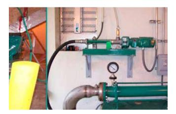
NETZSCH FLR System being used in conjunction with NEMO<sup>\*</sup> Sludge Cake Pump to convey dewatered sludge over 900 ft (275 m) for transport. With the introduction of only 0.7 gpm (.16 m<sup>3</sup>/hr) of polymer into the sludge, pressures are reduced from 450 psi to 150 psi (31 bar to 10 bar) for safe and easy long distance transfer within the pipeline. Sludge cake solids content approximately 23% being pumped at 20 gpm (4.5 m<sup>3</sup>/hr).
