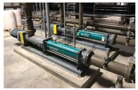
NETZSCH NEMO® 090 BY pumps in the Boiler Building transfer hydrolized food waste with extremely low pH product with 5% solids.
