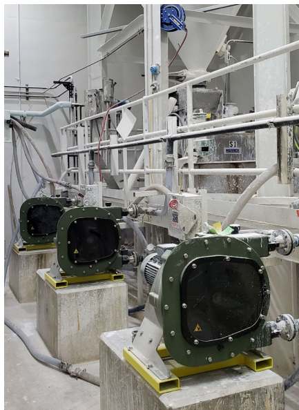
Three NETZSCH PERIPRO® pumps in series metering lime slurry for pH control at a Midwest water treatment plant.
